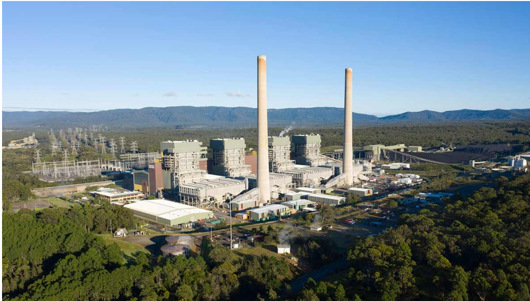
Central de carbón Eraring de Origin Energy, Australia
