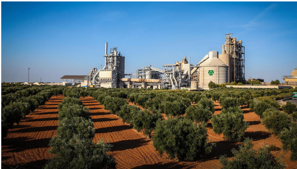
Fábrica de Cementos Portland.
