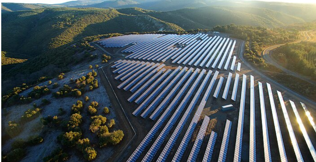
PV Project of Q ENERGY
